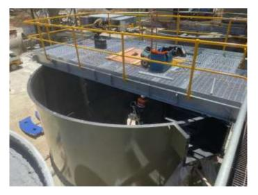
Image 2: New steel leach tank and agitator installation, underway
