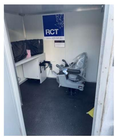
Image 3: New remote control room and associated systems for Kaiser's remote control mining equipment
