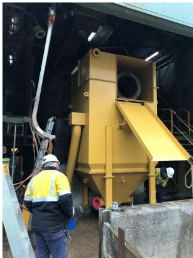
New discharge hopper installed in the SAG Mill building
