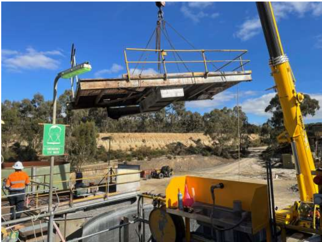
Old leach tank platform being removed
