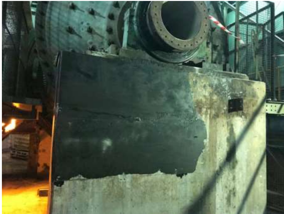
SAG Mill plinth/foundation repairs
