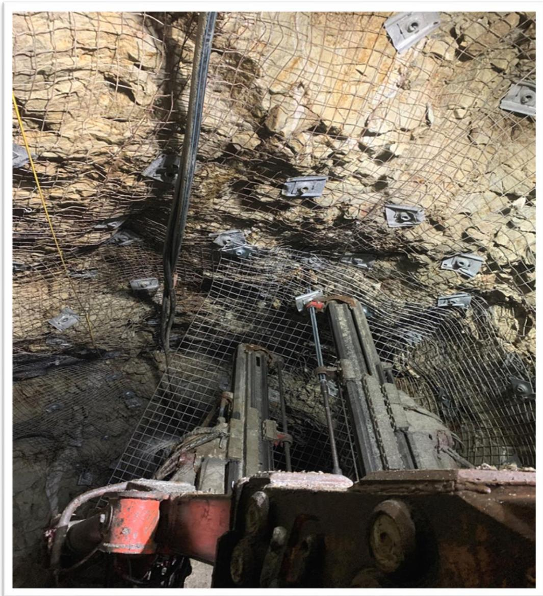
**Figure 4: Mesh and rock bolt installation in progress.**
