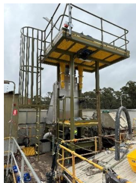
Figure 9 and 10. New Hydrocyclones
