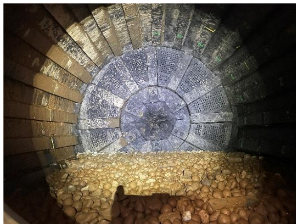
Figure 3. New Mill liners installed
