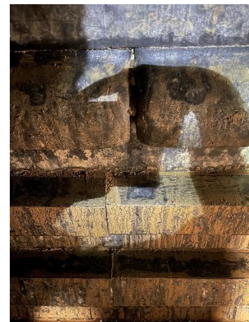
Figure 4. New and Old mill liners
