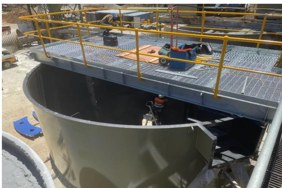
Figure 6: New steel leach tank and agitator installation, underway.
