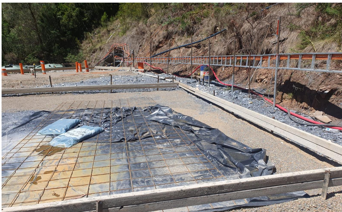
Figure 2: Generator and substation concrete pads awaiting concrete pouring and showing the orange HV cable conduits awaiting surface power generating equipment.
