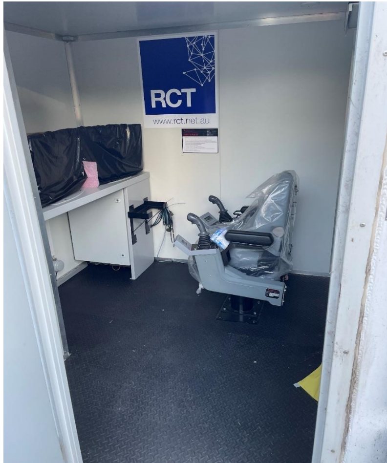
Figure 7: New remote control room and associated systems for Kaisers remote control mining equipment.
